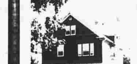
CONVENIENTLY LOCATED 3 Family, consisting of two - 5 room apts. and a 3 room apt., pantries, porches, 2 newer furnaces, 2 yr. old roof and 2 car garage. Don't wait on this one!
